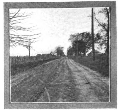
Showing a fine stretch of road near Lacolle after scraping
